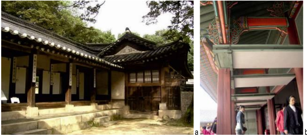
Figure 3: Traditional examples of structures with moving up doors: a) moving up doors in Changeoungkung palace. Source: www.geocities.com/asiaglobe/gallery ; b) moving up doors in Gyengbokgung palace. Source: author.
