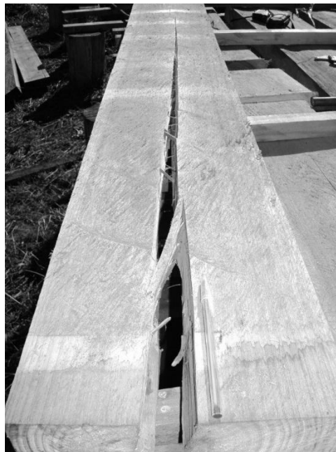
Figure 4. Juvenile wood plank of Eucalyptus grandis presenting a very long, deep and severe surface check.
