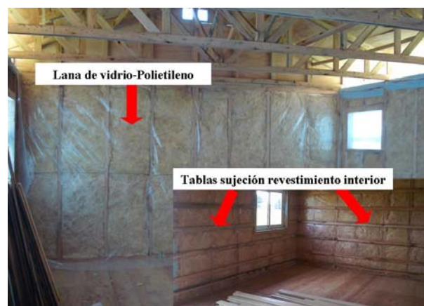
Figura 7. Aislamiento interno. Figure 7. Internal isolation.
