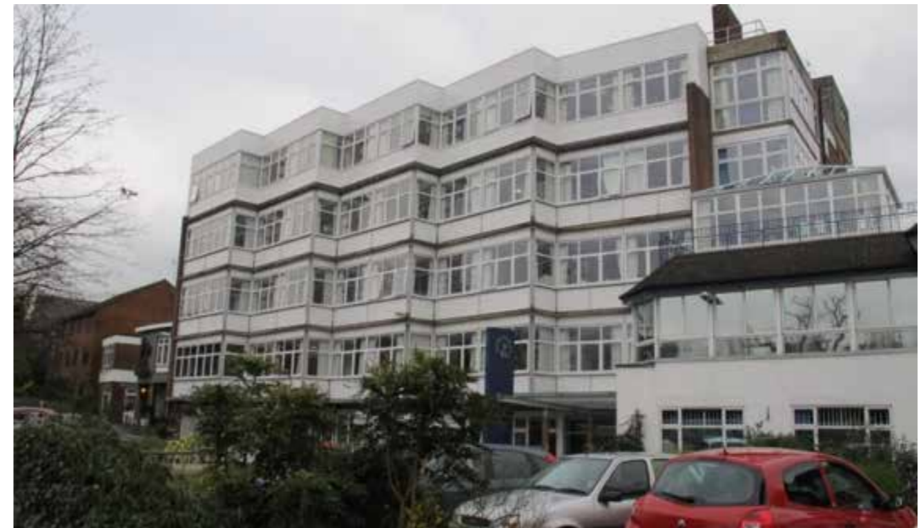
Figura 1 - St. Christopher's Hospice. Fonte: https://londonnewsonline.co.uk/hospice-reopens-shops-in-effort-to-plug-2m-funding-gap/
