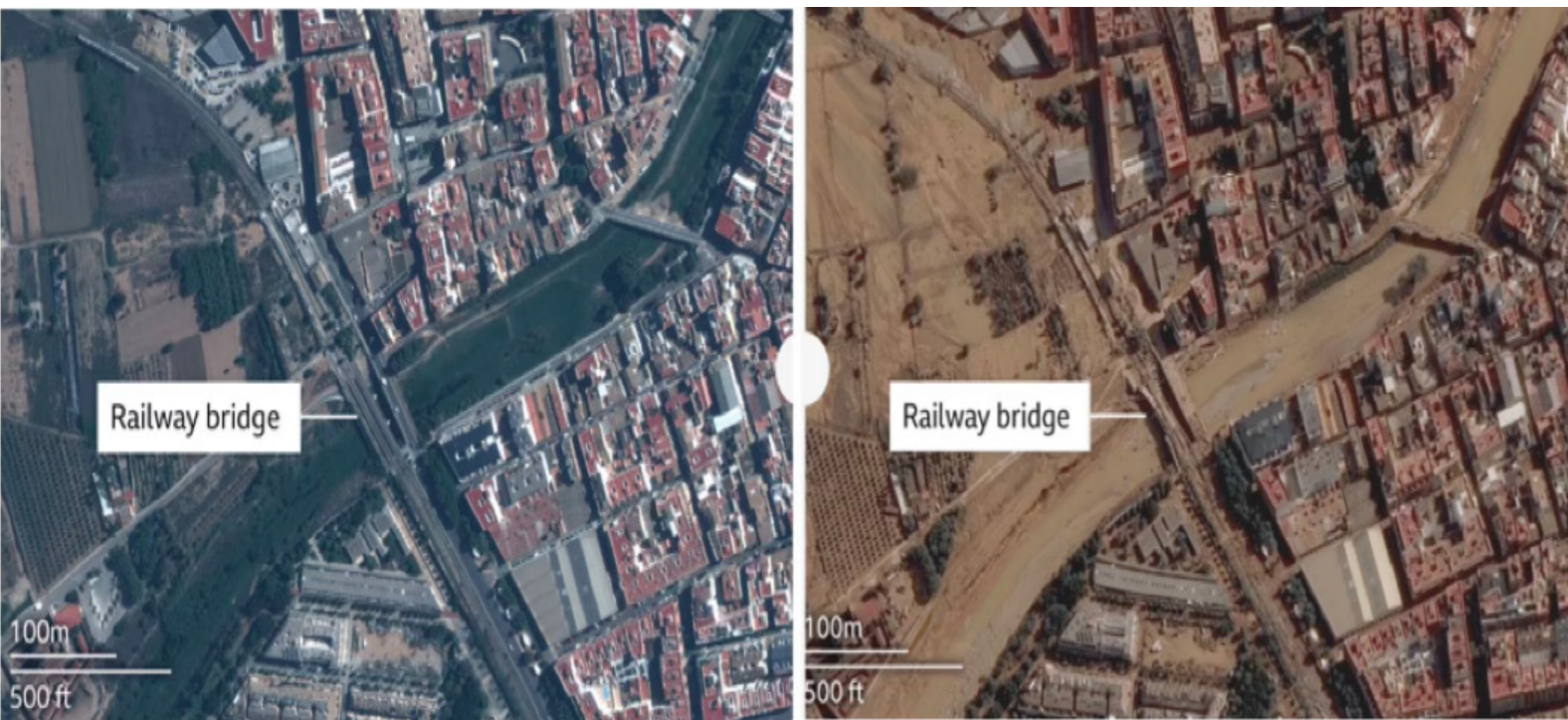
Figure 4 - Satellite imagery reveals the damage to road and railway bridges (before and after) caused by the Valencia floods. Dozens of meters of train tracks were destroyed. Service between Madrid and Valencia has been stopped until the lines are rebuilt (Source: BBC, 2024d). The floods destroyed homes and disrupted critical infrastructure like roads and railways, exposing vulnerability to environmental disasters.
