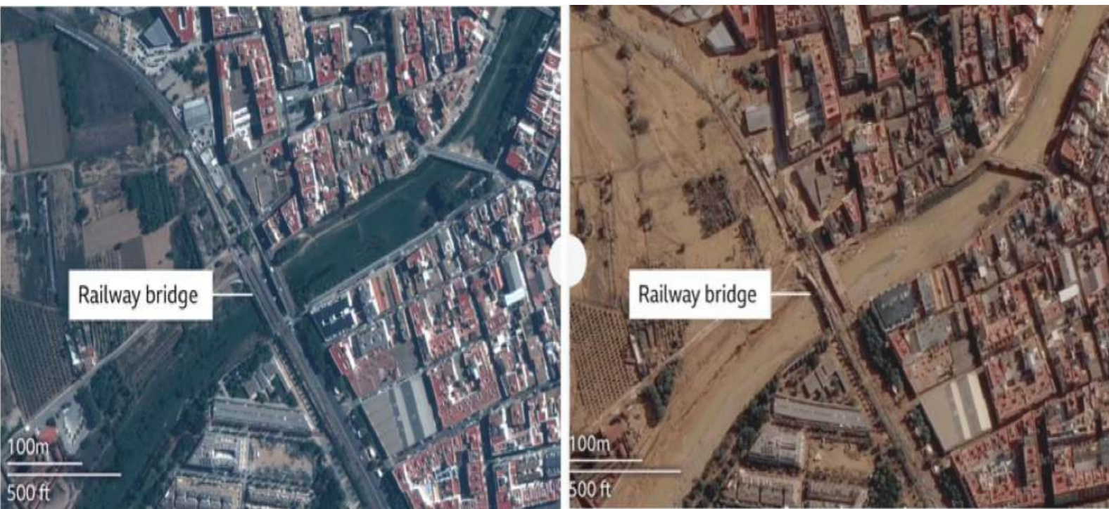
Figure 4 - Satellite imagery reveals the damage to road and railway bridges (before and after) caused by the Valencia floods. Dozens of meters of train tracks were destroyed. Service between Madrid and Valencia has been stopped until the lines are rebuilt (Source: BBC, 2024d). The floods destroyed homes and disrupted critical infrastructure like roads and railways, exposing vulnerability to environmental disasters.
